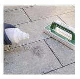
When the grout has hardened (after at least 7 days), any residue and streaks can be removed using **Fuga-Shock Eco**.
